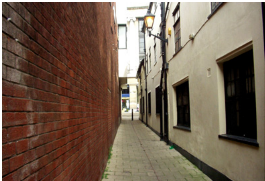
Figure 1: Historic alleyway within the City centre, near to the Old Market Square. This alleyway runs between St Peters Gate and the Poultry and dates back to c 1850's.
